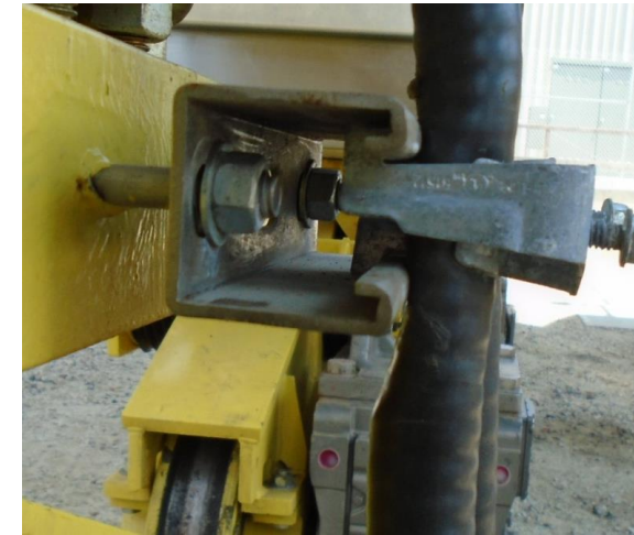
Figure 4—Example of cable tray with cable supported by rollers during pull
